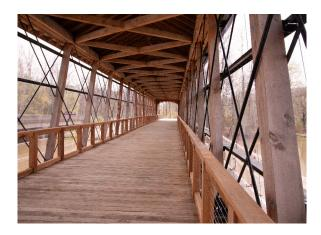
The Bell's Ford Covered Bridge was dedicated at Geist Park in Fishers, Indiana on September 5<sup>th</sup>, 202. It uses salvaged metal parts of the Post Truss that were salvaged from the former site of the Jackson County bridge. The sides of the bridge are plexiglass to allow the trusses to be seen when walking on the bridge.
